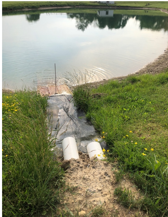
Figure 5. Polyvinyl chloride pipes (two 15.2 cm [6 in]) connecting the primary waste treatment pond to the secondary waste treatment pond.
