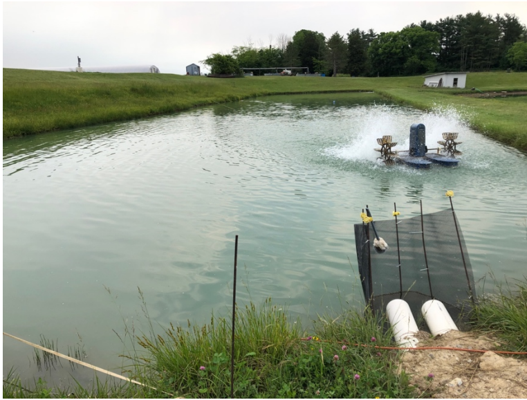
Figure 4. Polyvinyl chloride pipes (two 15.2 cm [6 in]) connecting the yellow perch culture pond to the primary waste treatment pond with a screen to prevent fish from escaping from the culture pond.
