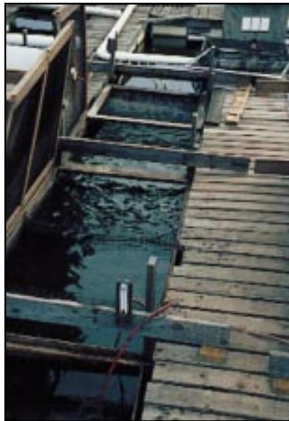
*Figure 1. IPR with dock—note blower housing and air-manifold are at the forward end of the raceway.*
