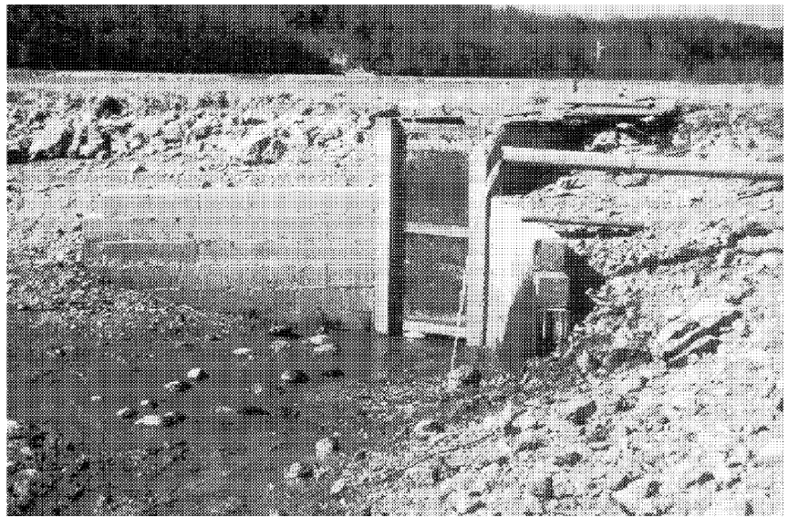
Figure 4. Pond at commercial fish farm with simple concrete monk that is built into the levee of culture pond. A supply of freshwater has been provided near the monk. Bumps in the catch basin are mostly turtles.
